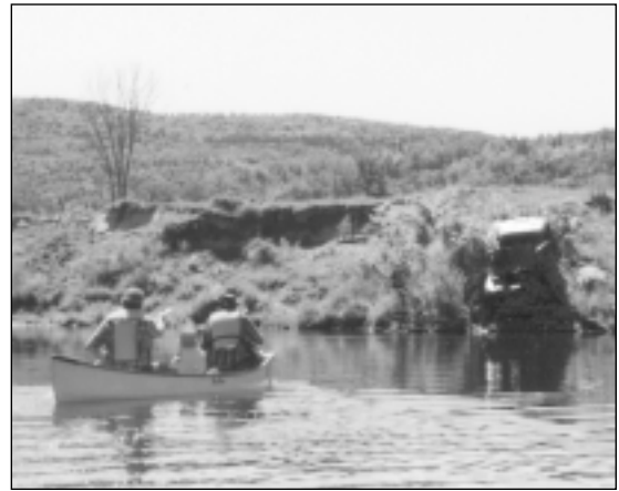
Erosion and vintage Detroit rip-rap in the Northeast Kingdom.
